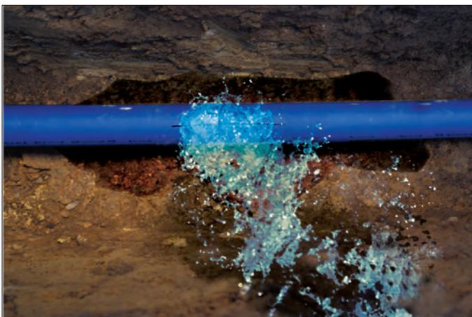
Typical longitudinal crack in a pipe typically caused by earth settlement or increased traffic load.
